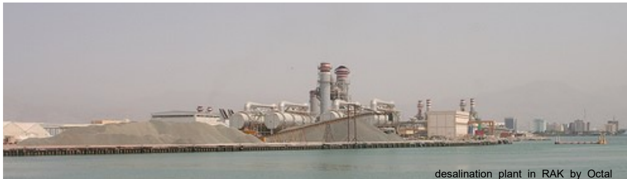
desalination plant in RAK by Octal
